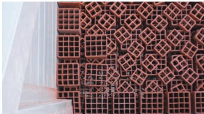
Tile fill as used in FM-approved cooling tower
