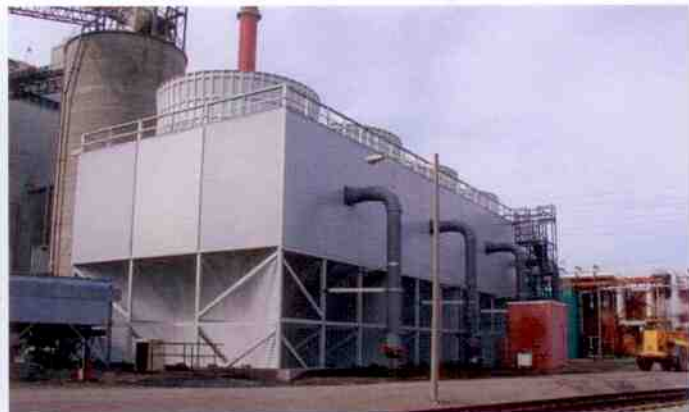
Due to high ambient temperatures, natural draught cooling isn't an option in the GCC.
