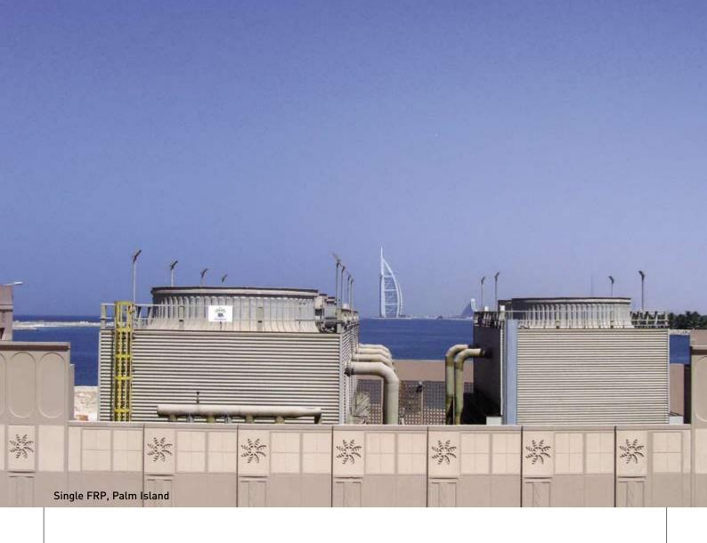
that each country seems to have its own preference in cooling towers. For example, the UAE appears to be partial to FRP cooling towers, while Kuwait seems to prefer concrete cooling towers. It is interesting to note that there are many examples of old and new towers that use ceramic tile file with a 25 year standard warranty on the fill, for both plant room size projects and small scale projects.
