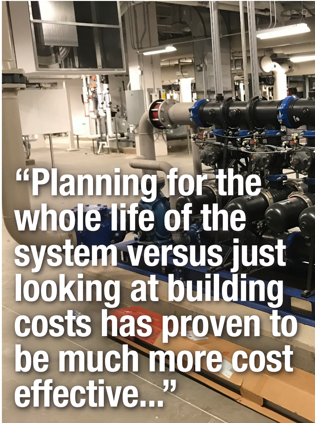
Cooling tower filtration comprises many different types of systems and options, including disc filters.
