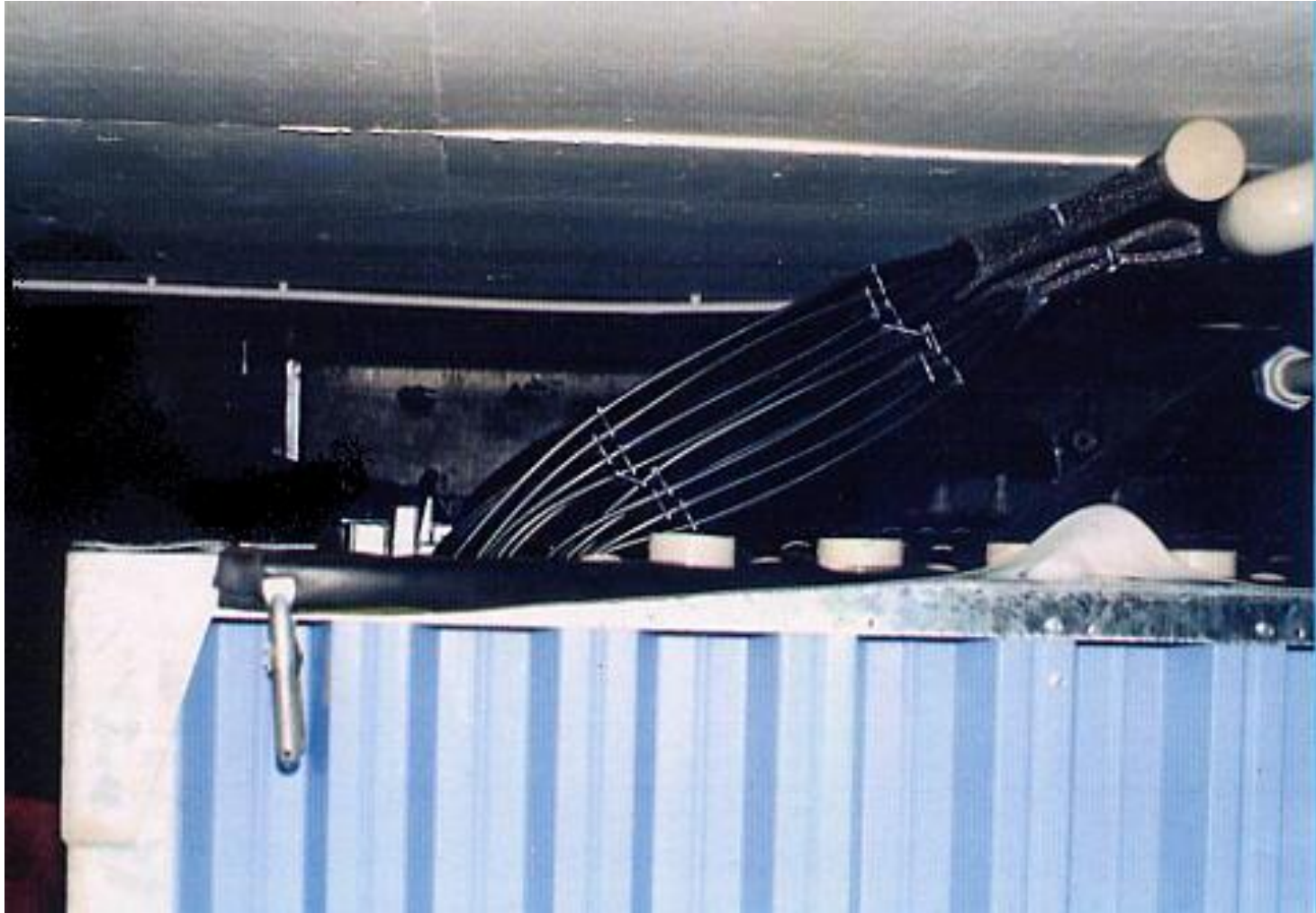
Installation of heat-exchangers
