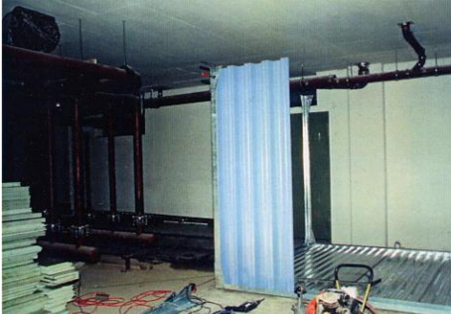
Assembly of trapezoidal wall sheets
