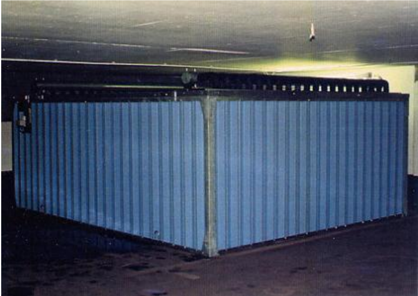
Ice bank ready for header insulation
