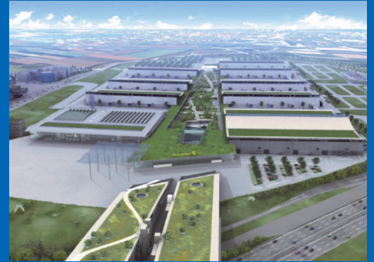
New Exhibition Stuttgart/Germany, Total storage capacity 56,000 kW-hr
