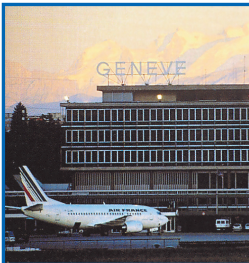
International Airport Geneva/Switzerland Total storage capacity 17,700 kW-hr
